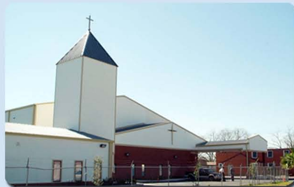
MT. VERNON BAPTIST CHURCH, HOUSTON TX.
